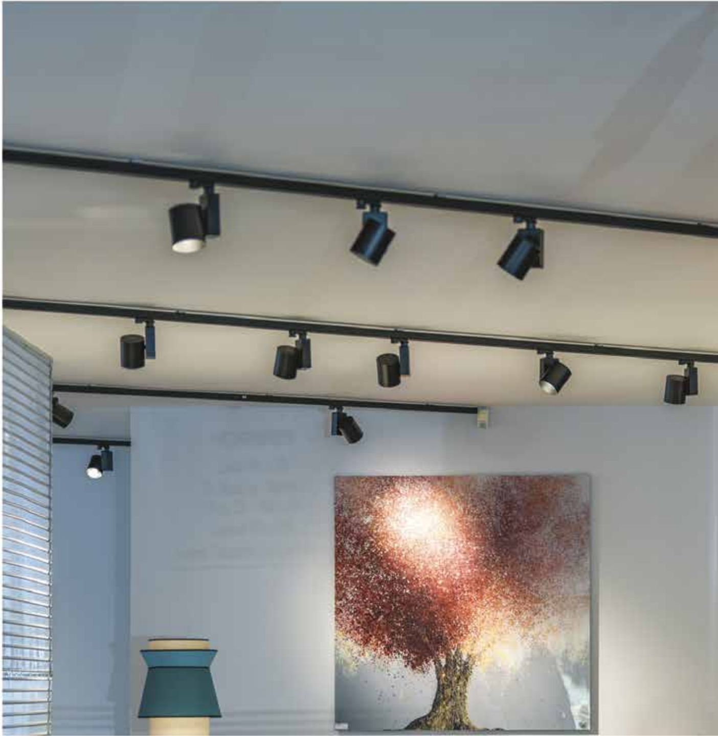
Cuir Center, Avignon, France Credit photo: Christophe Pozzo Di Borgo Lighting Design: LM5P, Aix en Provence, France
